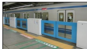
Maintenance of platform doors
