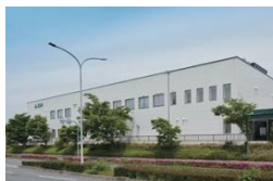
Kobe API Plant
