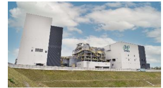
Currently under construction
