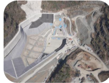
February 2022: Operation New controlled landfill site
