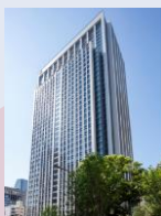
Kamiyacho Trust Tower
