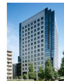
Osaki MT Building
