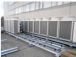
Renewal of air-conditioning system
