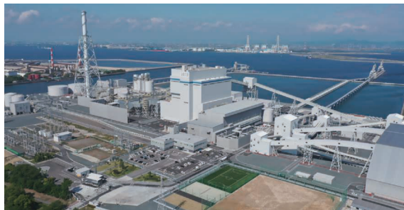
Taketoyo Thermal Power Station Unit 5, Civil Engineering & Building Construction Work (Chita-gun, Aichi)
