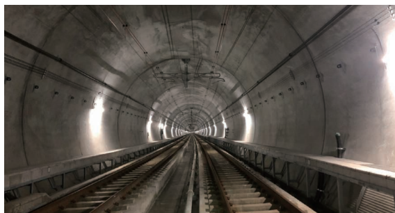
Hazawa Tunnel and Other Works for Sotetsu-Tokyu Link Line (Yokohama-shi, Kanagawa)
