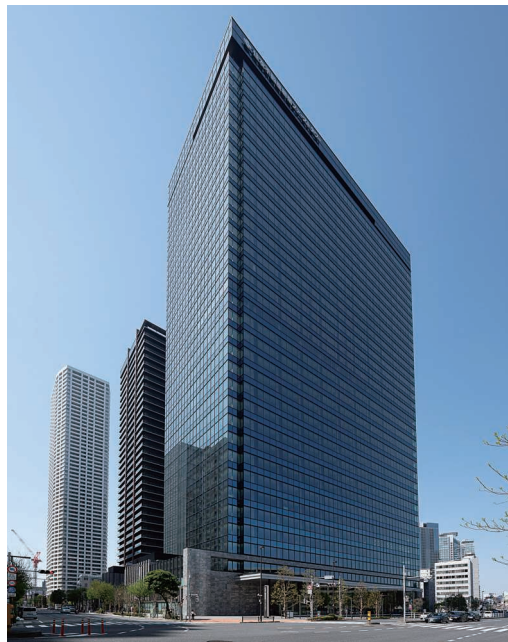
New Building Construction Work for Nishi-Shinjuku 5-chome Kita Project (Shinjuku-ku, Tokyo)
