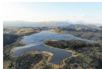
Oita Solar Power Plant (Oita Prefecture)
