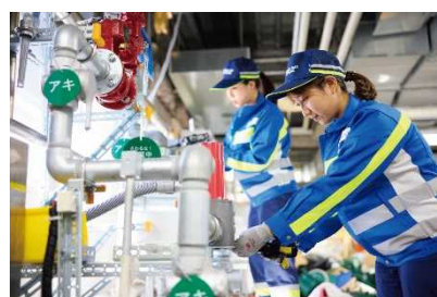
Safety inspection at a supply facility
