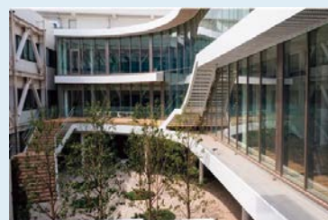
Tsukuba Research Laboratories after the completion of major renovations
