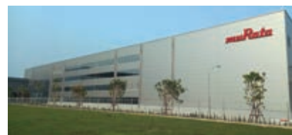
Murata Electronics (Thailand), Ltd.の新棟
