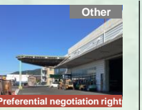
T&B Maintenance Center Matsue
