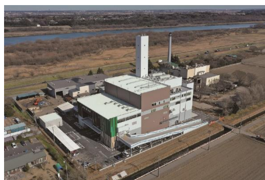
Abiko Clean Center, Chiba Prefecture
