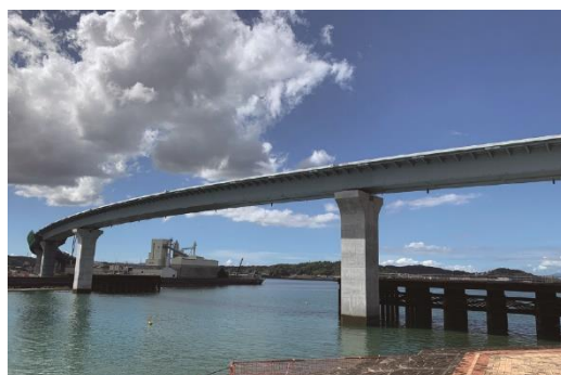
Amakusa Mirai Bridge (Kumamoto Prefecture)
