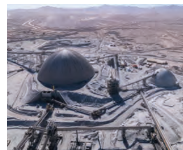
Centinela Copper Mine (Chile)
