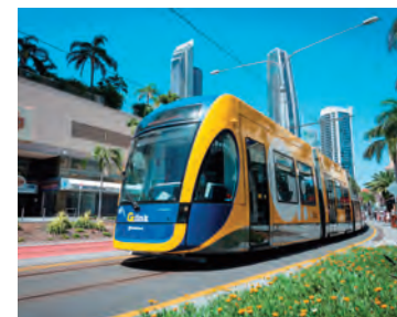
Extension project for Gold Coast Light Rail (Gold Coast, Australia)
