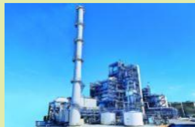
Tokuyama Biomass Power Plant
