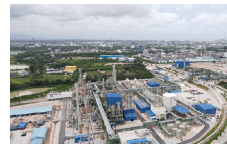
Aerial view of the new plant
