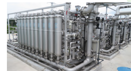
GL module units installed at Kurashiki Plant
