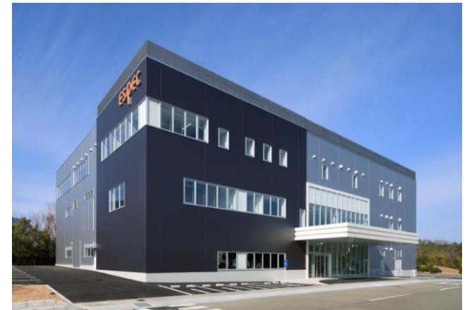
Technology development building
