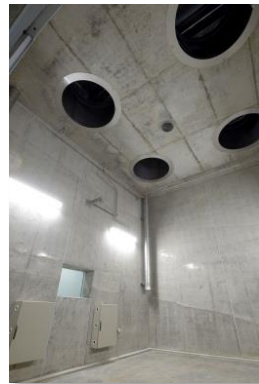
No. 2 Safety Test Room
