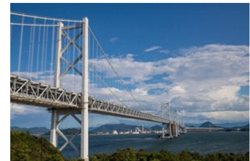
Kita Bisan-Seto Bridge and Minami Bisan-Seto Bridge
