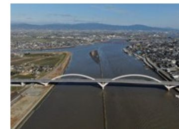
Ariake Chikugo River Bridge The first bridge of its type in Japan Japan Society of Civil Engineers "Tanaka Award"
