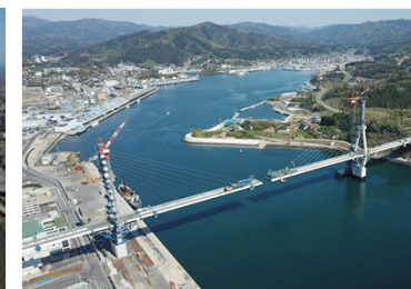
Kesennuma Bay Crossing Bridge (1,344m) A symbol of Japan's recovery from the Great East Japan Earthquake Japan Society of Civil Engineers "Tanaka Award"
