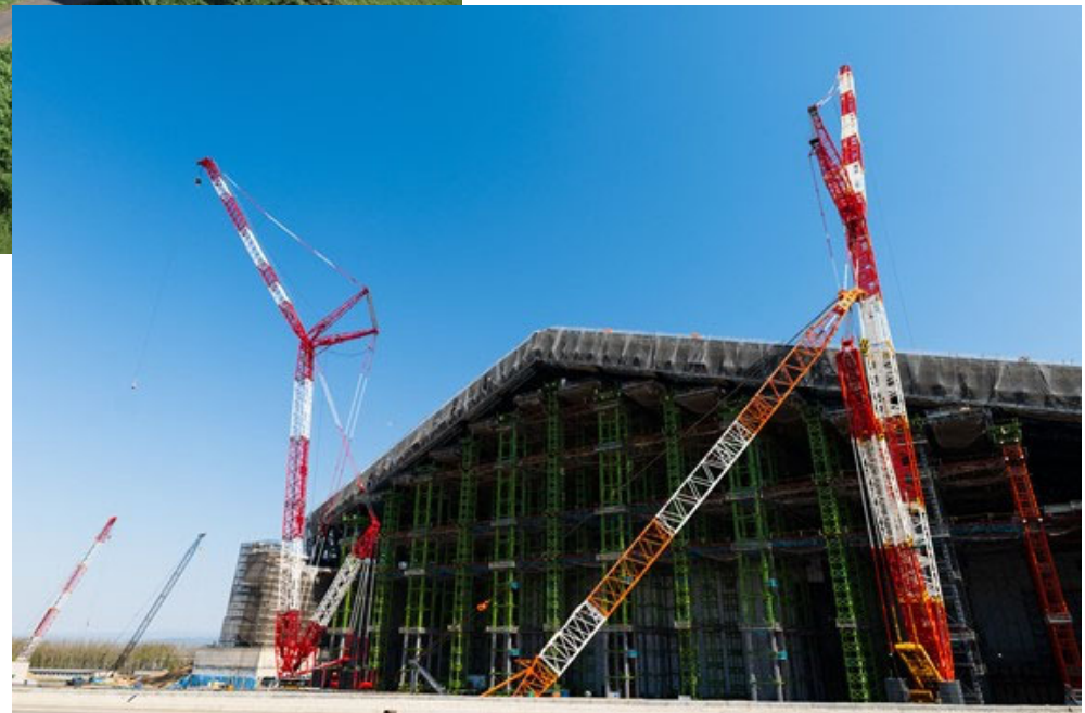
Hokkaido Ballpark steel frame OBAYASHI CORPORATION and other JVs
