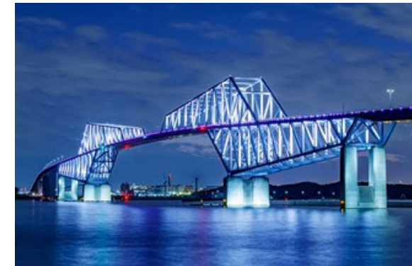
Tokyo Gate Bridge (2,618 m) Japan's second-largest truss bridge Japan Society of Civil Engineers "Tanaka Award"
