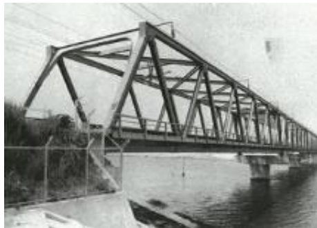
Tokaido Shinkansen Egawa Bridge
