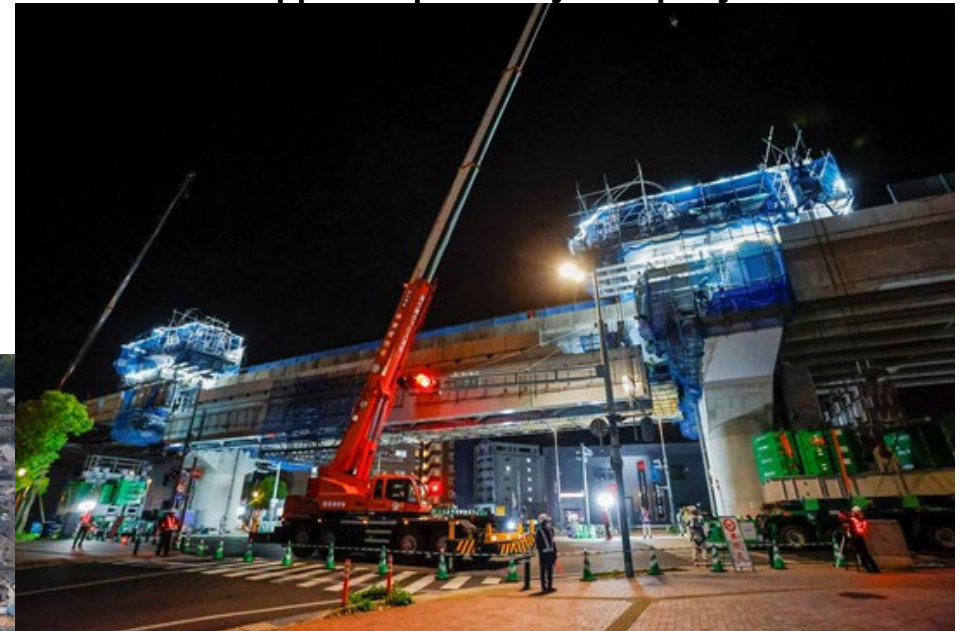
Sasebo Viaduct widening – West Nippon Expressway Company Limited
