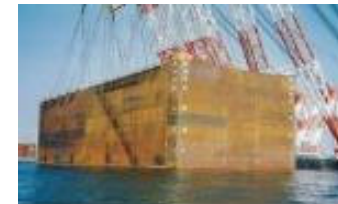
Minami Honmoku steel caisson
