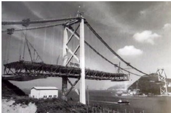
Kanmon Bridge (1,068 m) Erected using the pioneering successive rigid coupling technique Japan Society of Civil Engineers "Tanaka Award"
