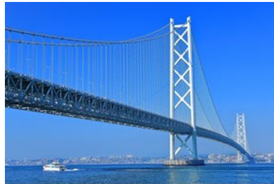
Akashi-Kaikyo Bridge (3,991 m) The world's largest suspension bridge at the time of its construction Japan Society of Civil Engineers "Tanaka Award"
