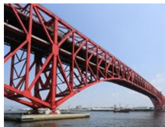
Minato Bridge Japan's largest truss bridge Japan Society of Civil Engineers "Tanaka Award"
