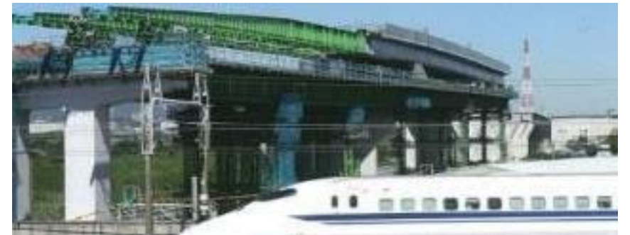
Sagami Jukan Expressway No. 16 Bridge near the Tokaido Shinkansen 50K900 point
