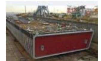
Tokyo Bay Umi-no-Mori Tunnel immersed tube tunnel
