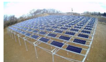
Yabuki Town Solar Sharing Power Plant
