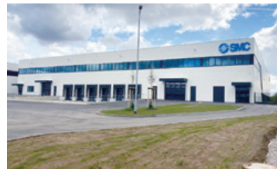
SMC Germany Production facilities/warehouse (Hessen, Germany)
