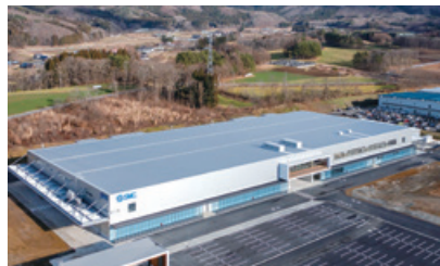
Tono Factory No.2 (Tono-shi, Iwate prefecture)
