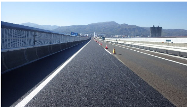
Sasson Expressway Hassamu Viaduct floor slab waterproof work
