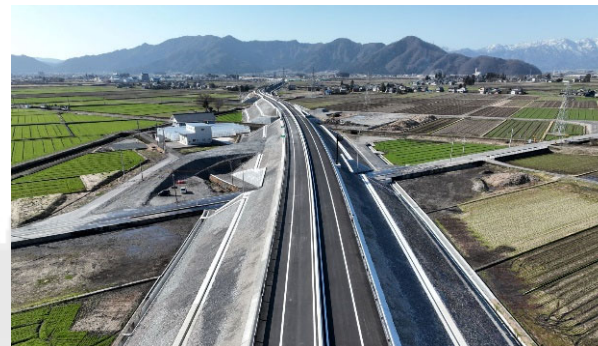
Pavement and other work in Tano area on Ono Aburazaka Road
