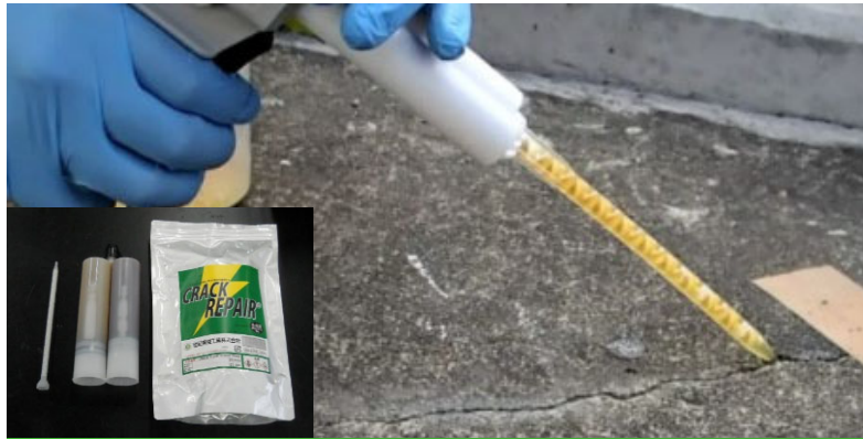
CRACK REPAIR
