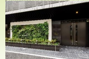
GENOVIA Higashi-Nihombashi Ekimae green veil
