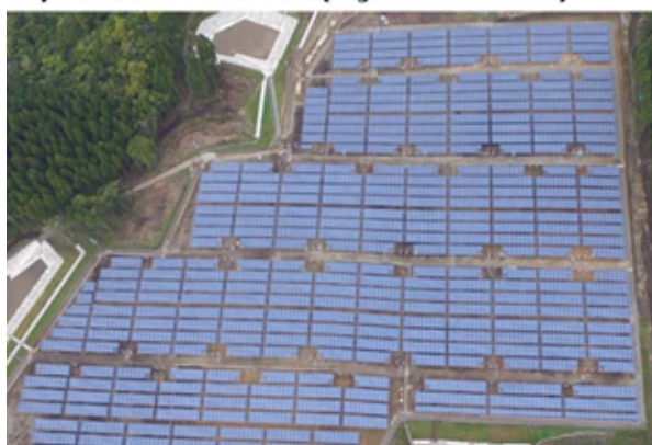
Miyanoura Solar Power Plant (Kagoshima Prefecture)
