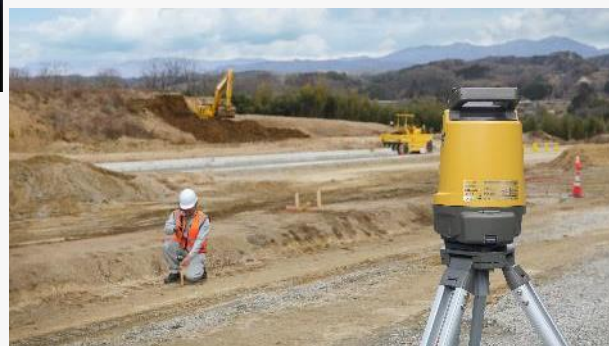
Layout Navigator LN-100 at Construction site
