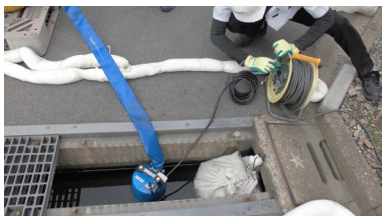
Tamamura Plant We conducted shielding and collection training for drainage ditch assuming that a chemical substance leaked into the drainage ditch. (August 2022)
