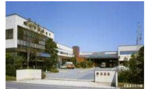
Kotobuki Seika Co., Ltd., Main Plant
