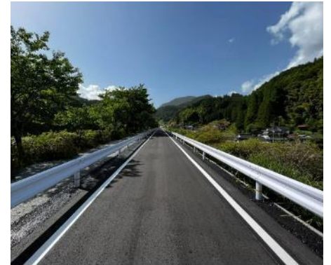
JR Kyushu's bus rapid transit (BRT) dedicated road paved with NEWTLAC
