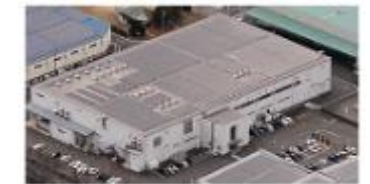
Japan (Toyohama Manufacturing Site)
