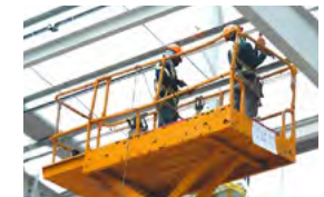
Aerial work platform at construction site
