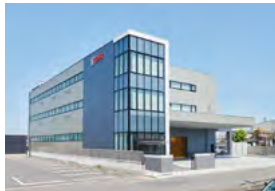
Renovated head office (top) and factory (bottom)
