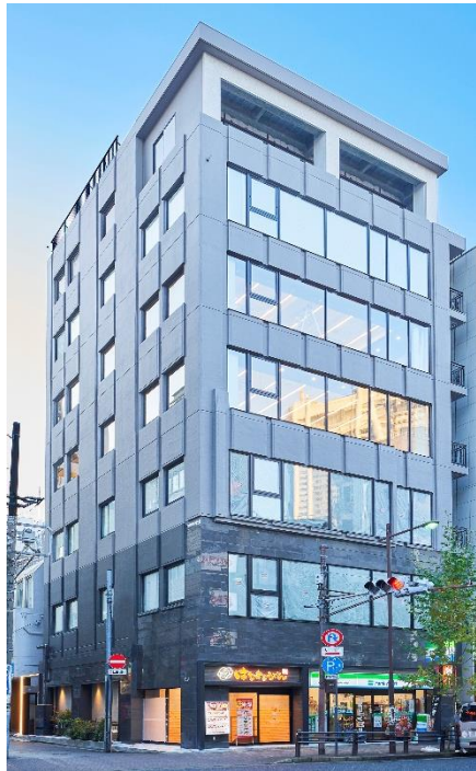
[Building appearance (after replanning)] Kandamisaki-cho, Chiyoda-ku, Tokyo Steel-framed reinforced concrete, 7 stories high with 1 basement
