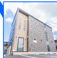
Tabino Hotel live Sado Start operating in June 2023
