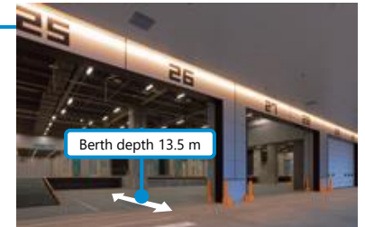
Truck berths are large enough to fit a whole 40ft container truck.
