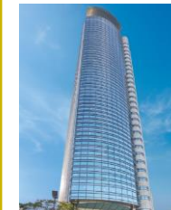
Nakanoshima Mitsui Bldg. (Osaka City, Osaka)
