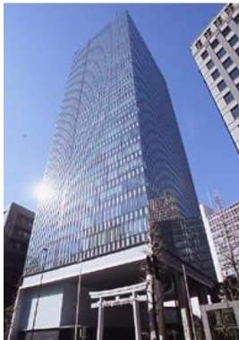
Toranomon Kotohira Tower: Project to Preserve a Tokyo Metropolitan Government Selected Historical Building (Kotohiragu) and Harmonize with the Shrine Grounds and Approach
