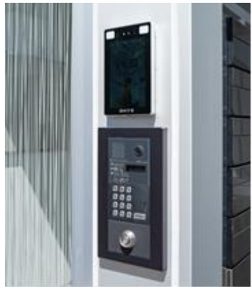
Face recognition system installed at entrance
