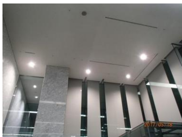
Shinagawa Seaside Parktower (Entrance)
