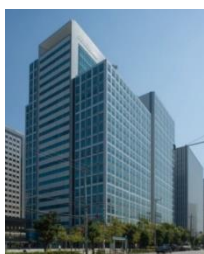
Shinagawa Seaside Parktower
