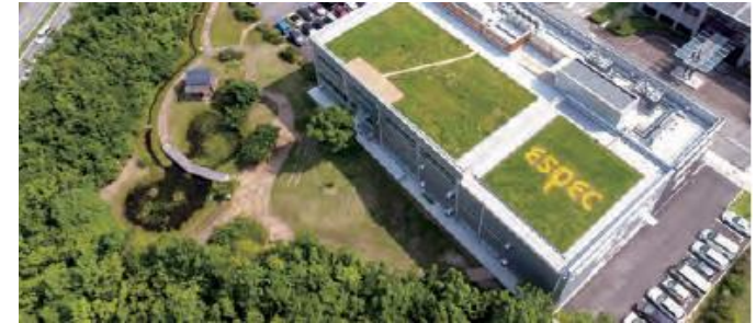
Rooftop green space using native species
