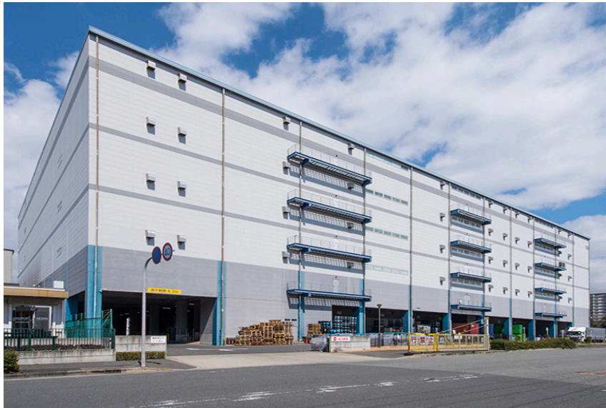
MJ Logipark Osaka 1
