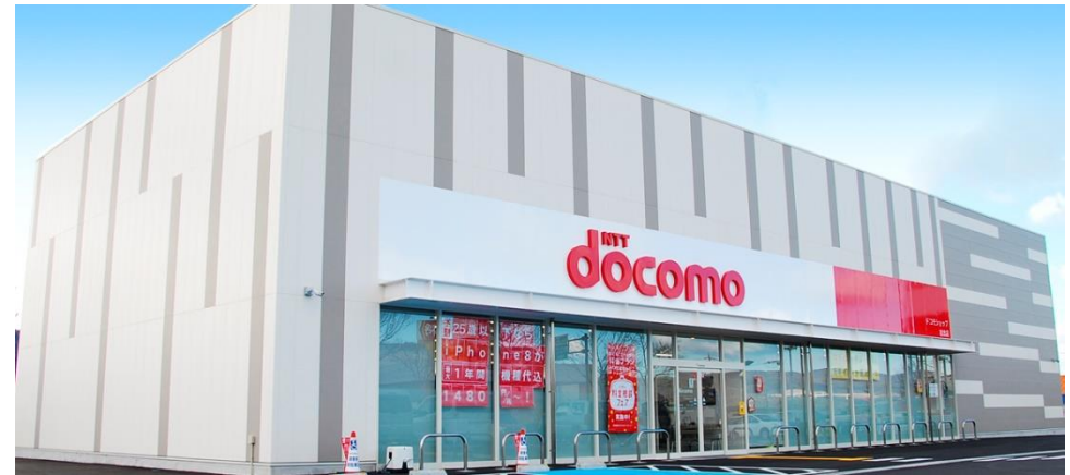
Iwade Store (largest store in Wakayama Prefecture)
