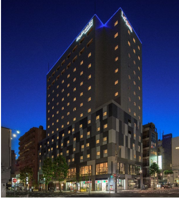
Appearance of Building
