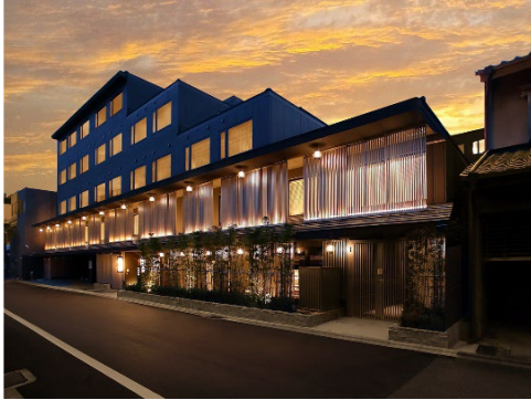
Appearance of Building
