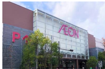
Exterior wall painting
