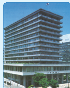
Former Nippon Credit Bank, Ltd. Head Office
