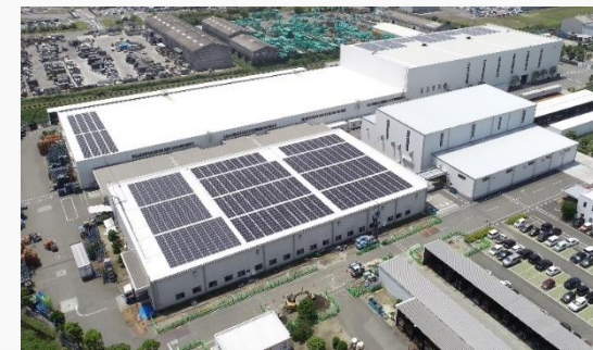
< Front > Logistics building < Back > Plant building
