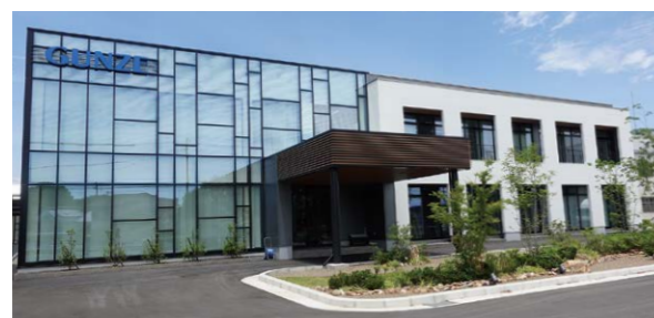
New ZEB certified office (Konan Plant)
