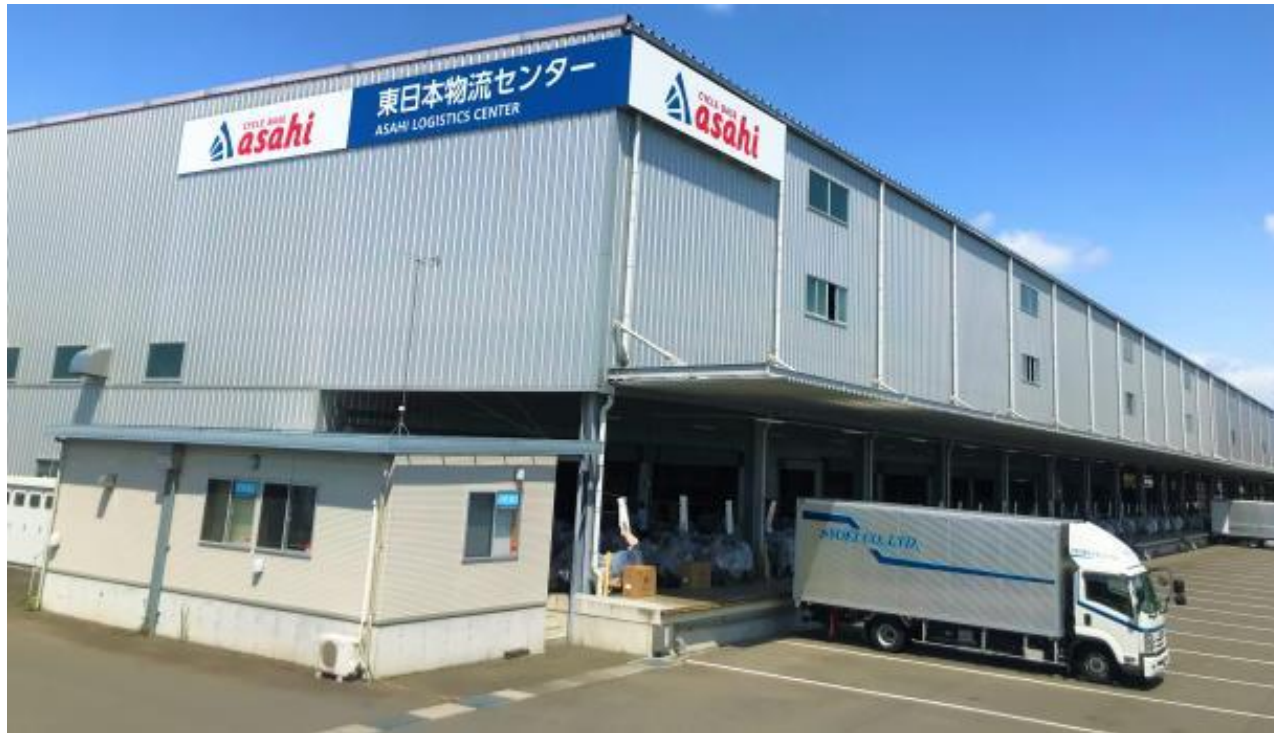
ASAHI warehouse at East Japan logistics center (Saitama)
