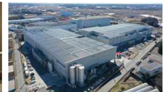
In Kanto Yachiyo area, where there is a cluster of six plants, three logistics facilities, and one recycling-related facility, we began operating solar power generation facilities in March 2022. We also began operating such facilities in the Chubu area in October 2022.
