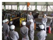
Demonstration of actual lifting operation
