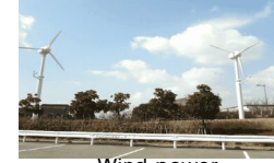
Wind power generation
