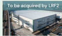
To be acquired by LRF2 Osaka Suminoe Logistics Center Completed in Mar. 2023
