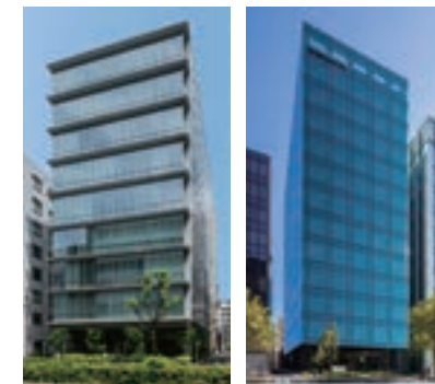
Keihanshin Onarimon Building (Completed in 2009)
