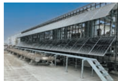
Solar panels on the Keihanshin Fuchu Building
