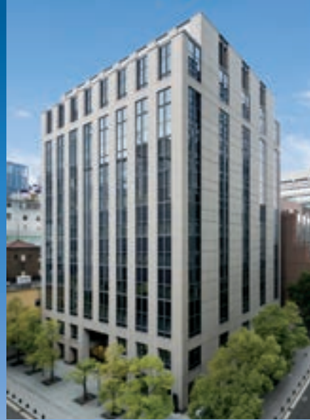
Keihanshin Yodoyabashi Building
