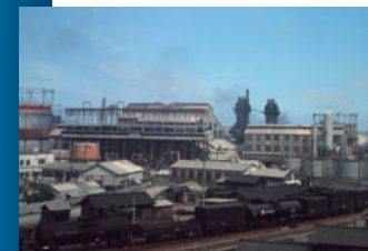
1952 Methanol manufactured from natural gas
