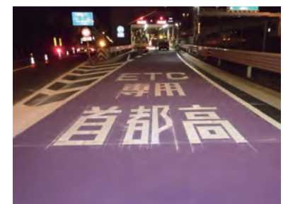
Dedicated ETC lane marking on the Metropolitan Expressway
