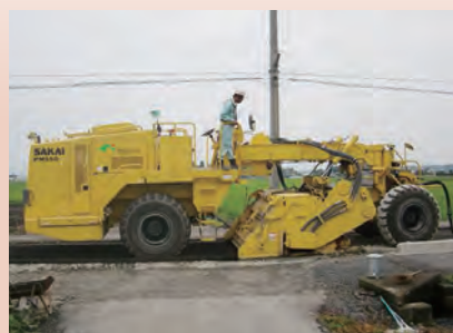
On-site base course recycling construction method STABI-CEMENT RC construction method
