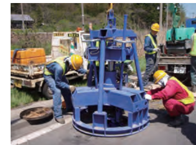
During construction (removal of a manhole)
