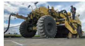
Construction with a road stabilizer
