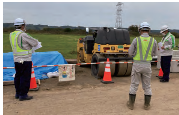
On-site safety patrol
