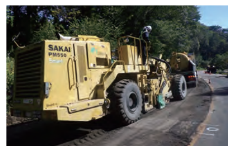
STABI-CEMENT RC construction method using ICT
