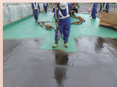
High-performance bridge deck waterproofing method HQ HIBRANE AU construction method
