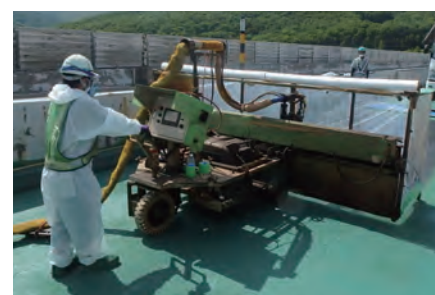
HQ HIBRANE AU construction method using a binder spraying robot
