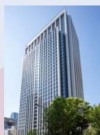
Kamiyacho Trust Tower
