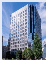
Osaki MT Building
